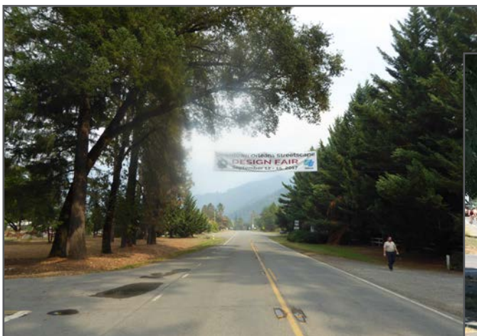
Figure 2: Highway 96 Lacks Adequate Shoulders
