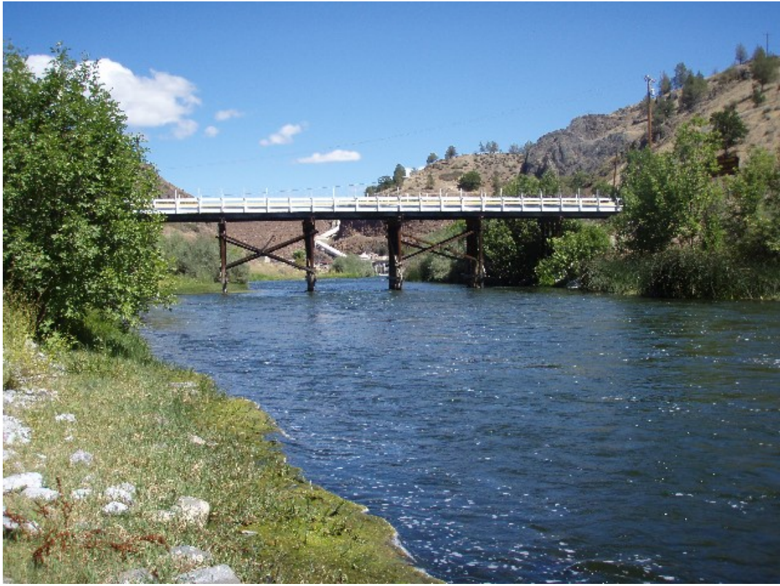
Figure 2 - Klamath River below Iron Gate Dam across river looking up from water quality station.
