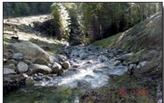
After Road Stream Crossing Excavation
