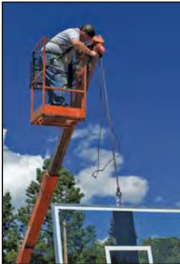
Tribal volunteer Ron Parton on lift raising heavy poles/backboards
