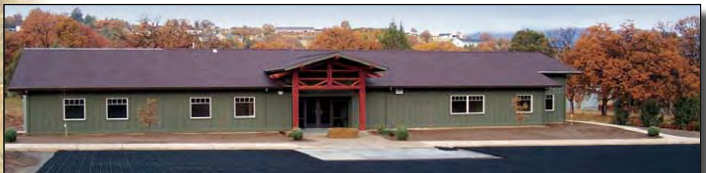
Newly completed KTHA/KTOC Community/Administrative Building
