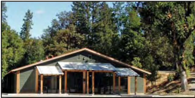
Happy Camp Senior Center (Former Headway building)
