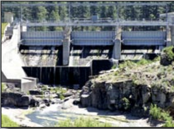
JC Boyle Dam, One of Four Dams Targeted for Removal on Klamath River
