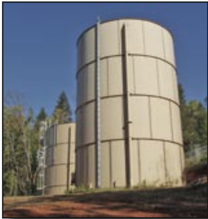
Water storage tanks above Karuk Tribal Housing in Happy Camp
