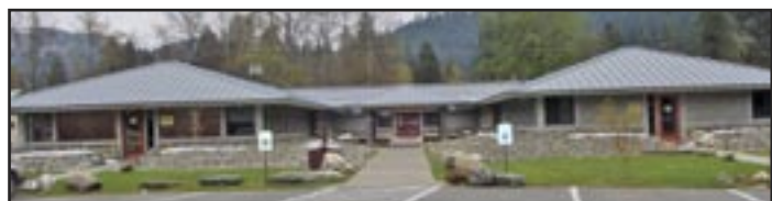
Administration Building, Happy Camp
