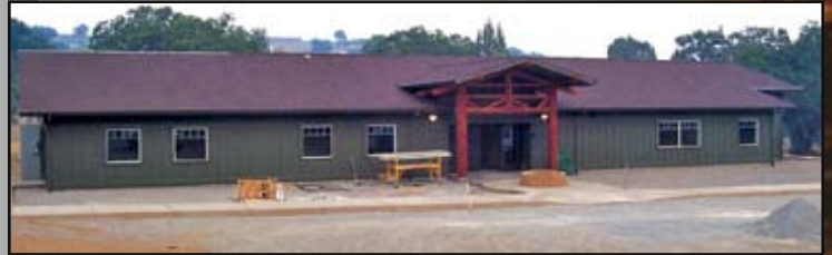
Newly Completed Yreka facility built in time for the August Council meeting
