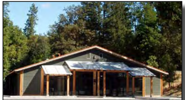
The Karuk Community Building which houses an office for the KCLF is located at Highway 96 & Second Avenue in Happy Camp
