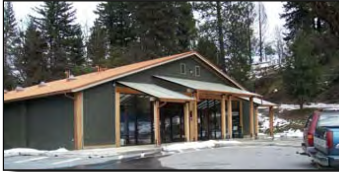
Above: The Karuk Tribe Housing Authority completely renovated the old Headway building in Happy Camp. It now houses the Senior Center, Council Chambers, Tribal TANF and Karuk Community Loan Fund offices
