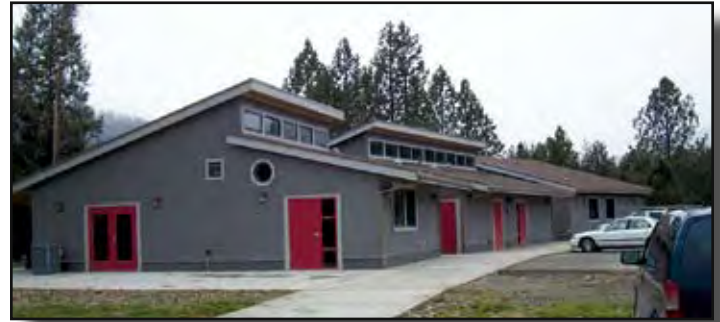
Newly Built Panamnik Center in Orleans
