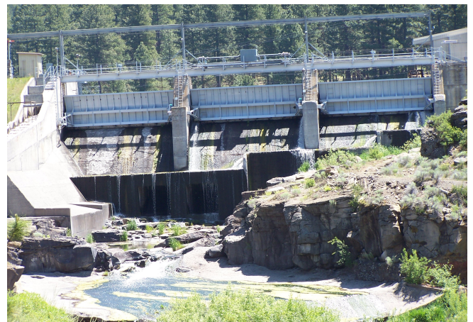
J.C. Boyle Dam diverts the majority of the river's flow through a mile of flume (photo courtesy of Steve Pedery)
